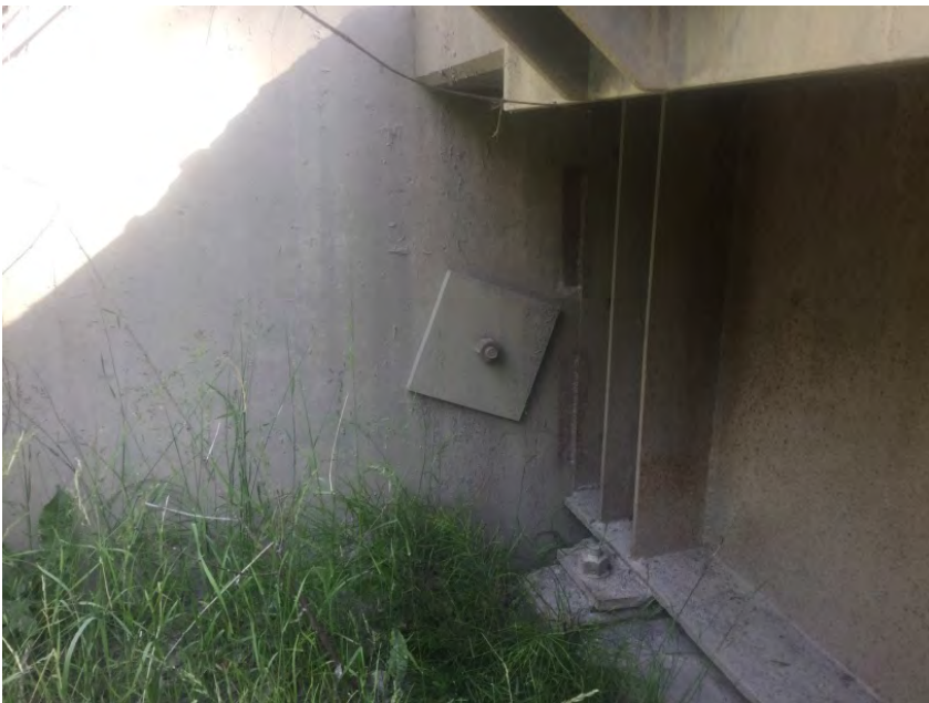
Ballast walls tieback system, typical both walls
