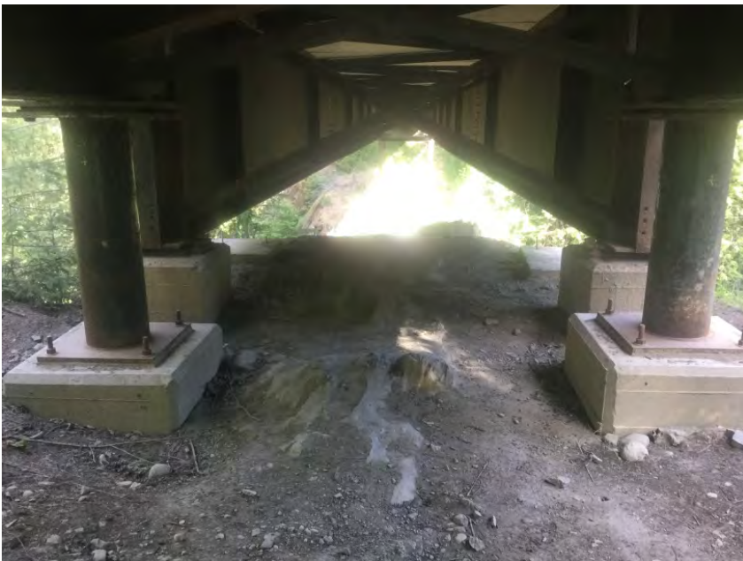
Main span left abutment and right span left abutment
