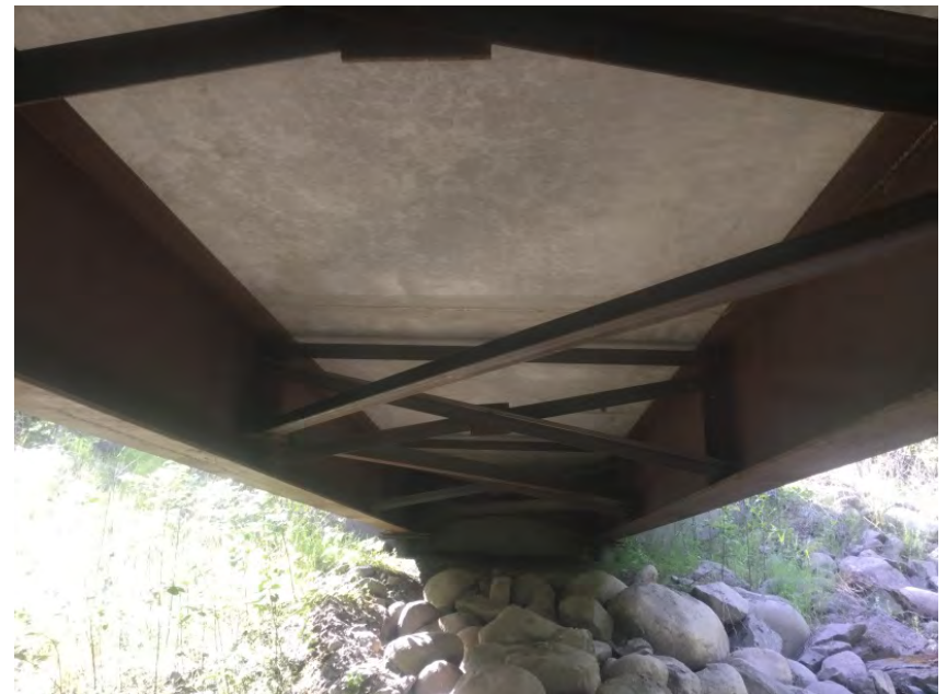
Right span superstructure
