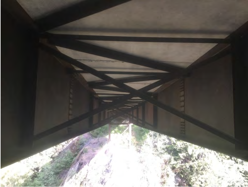
Main span superstructure
