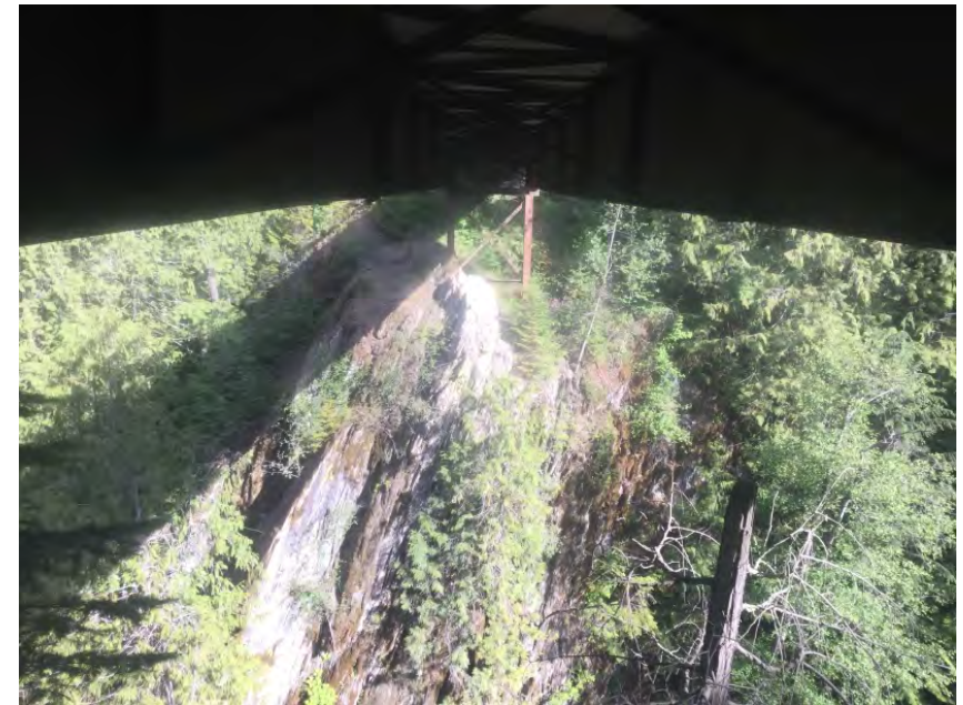
Left Bank Abutment when facing downstream
