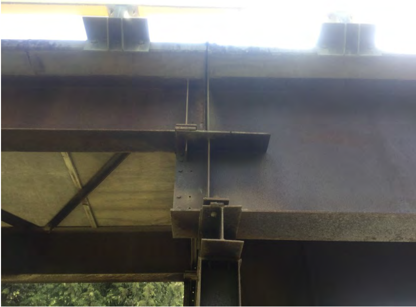
Left span to main span connection
