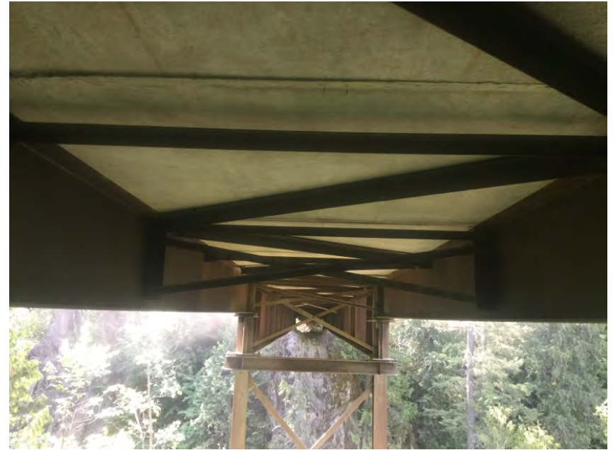
Left span superstructure
