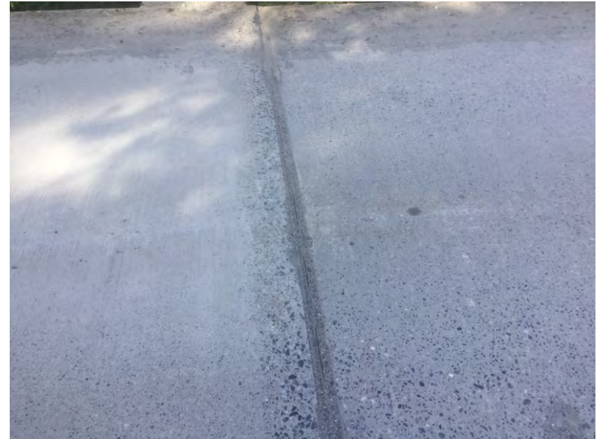
Right span to main span deck seal in place and functional
