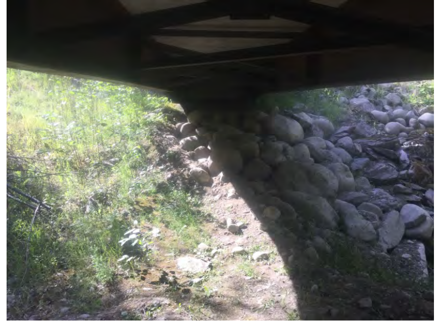
Right Bank Abutment when facing downstream
